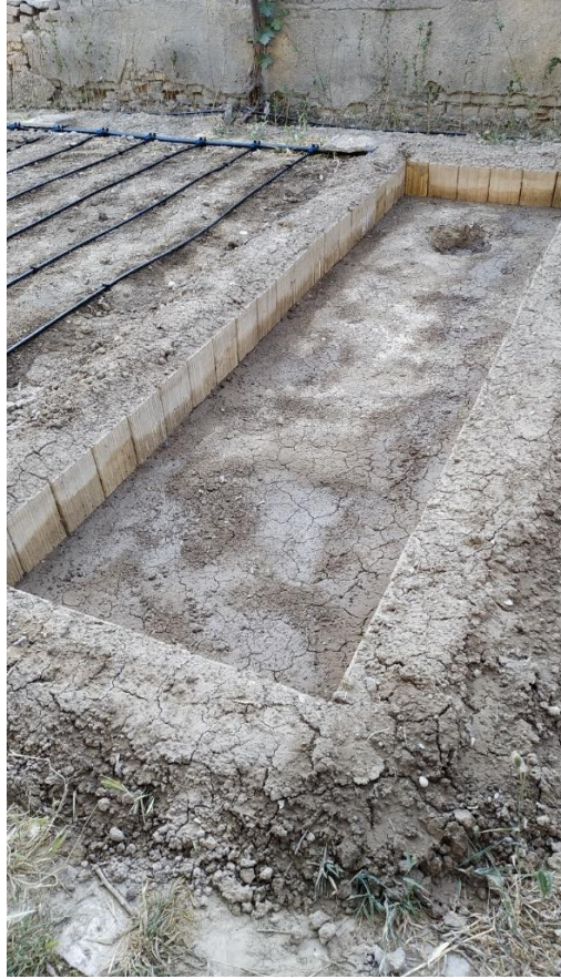
Figure 4: Floating Raft System Reservoir
