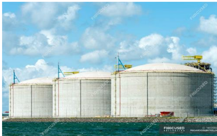
Figure 2-Huge tanks for LNG in the Rotterdam harbor.
