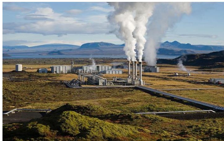
Figure 6-Geothermal power plant (flash steam, combined cycle) in Iceland.
